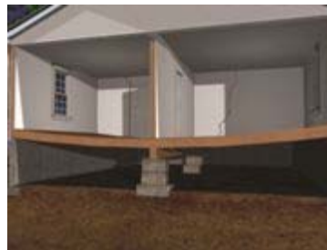
Sloping Floors caused by sagging girders and floor joists.
